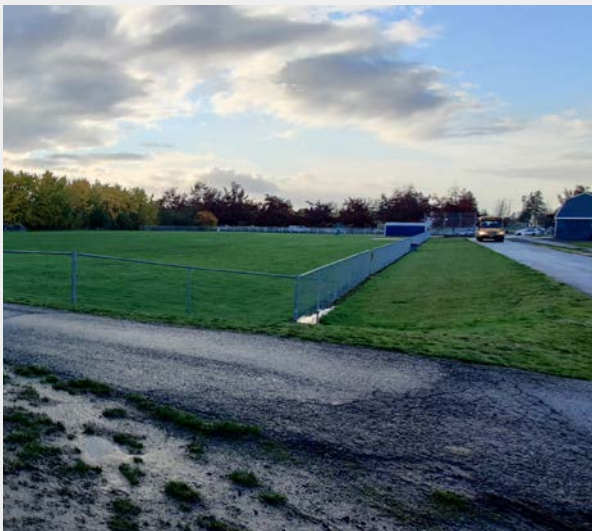
At the north end of the District-owned access driveway, another paved shared-use path connects to the Arbor Village neighborhood to the east.
