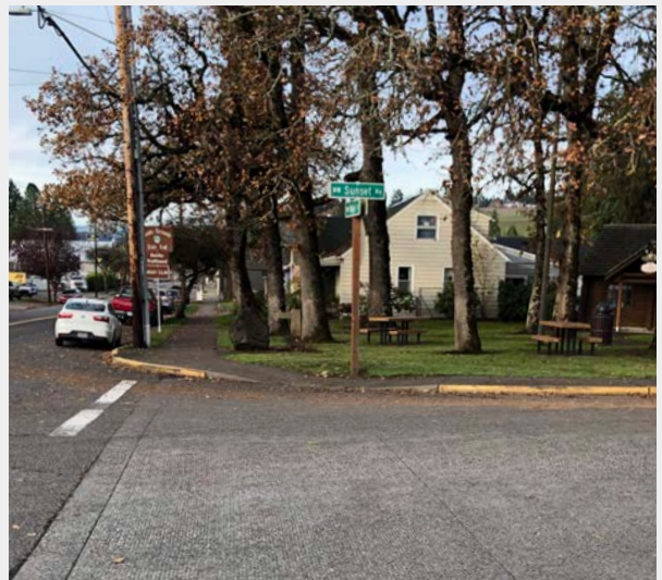
At Sunset St and Highway 47, the stop bar has been painted in front of the curb ramp, increasing the likelihood of potential conflict between vehicles and pedestrians.
