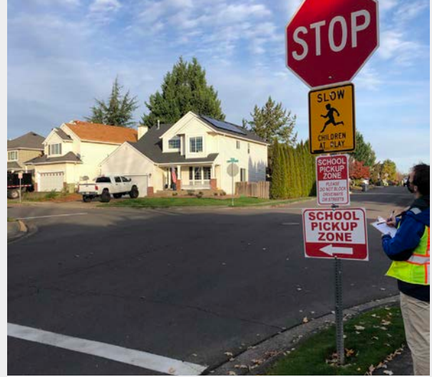
Although Devonmoor Ave and Oak Way is a four-way stop and there are curb ramps at all four corners of the intersection, no crosswalks currently exist across any of the approaches.
