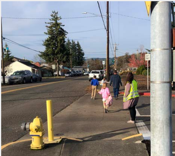
The sidewalk ramps at the entrance and exit of the High School and Middle School parking lot present wide crossing distances and are not ADA compliant.
